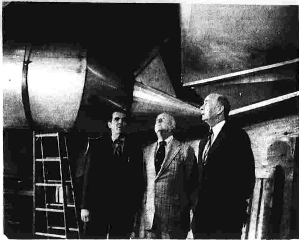
An air-to-air heat reclamation system in Manchester Memorial Hospital's new laundry is being inspected by Edward M. Kenney, left, hospital administrator, Robert J. Smith, president of the hospital's board of trustees, and John S. Murtha of the Hartford Foundation for Public Giving. (Herald photo by Pinto)
